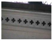
the windows on both side of the church are really decorative grilles for heating pipework which was small bore high temperature steam heating (very noisy due to expansion).
